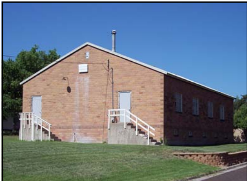
BACK VIEW of the building
