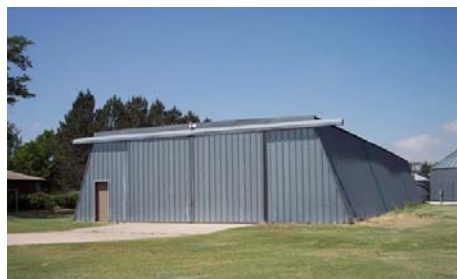
50'x125' Metal Building
