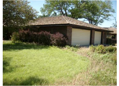
View of Attached Garage
