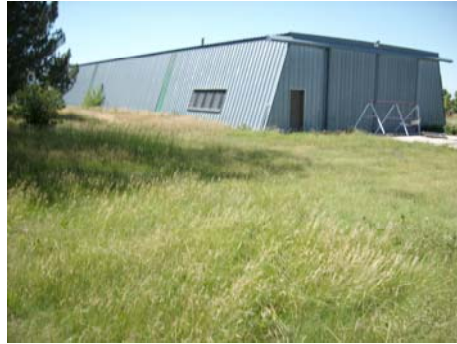
50'x 125' Metal Building
