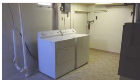
Basement Laundry Room
