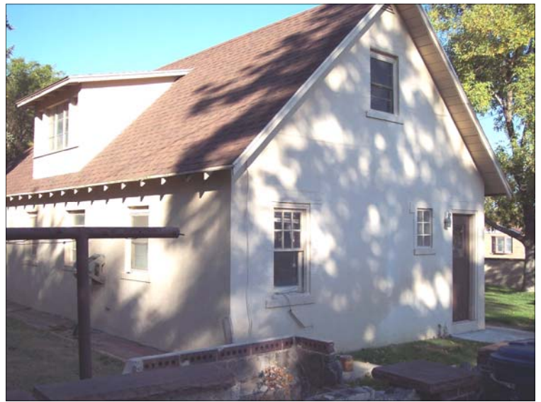
View of Garage from East
